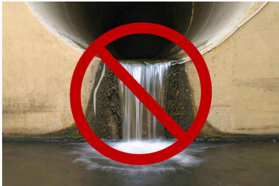
Figure B-1 Do not install LaserFlow Ex with built-in sensor in a free-flowing outfall or in a drop manhole.
